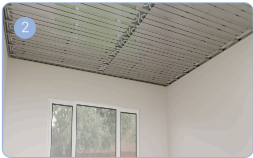
INNSJO ceiling panels installed within the ceiling structure.
