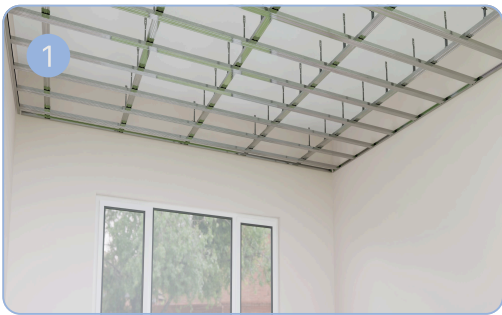
Cross-suspended ceiling structure.
